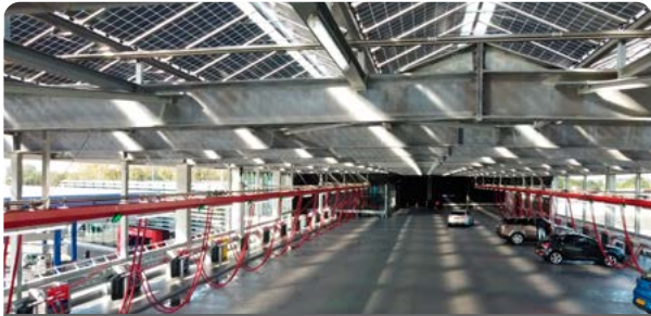
station de lavage
